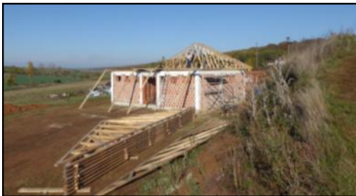
Building the Hygiene Centre
